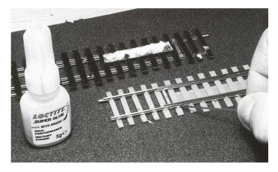
I peel the templates and the double-sided tape off very, very carefully - especially around the switch area, which is vulnerable because the slide chairs don't physically grip the rail, they're only there because they're clipped into the web. For extra insurance I always leave a little bit of tape on the back of this area while I'm still playing around with the turnout. Any chairs that look as though they're in danger of dropping off can be fixed with a drop of cyano or even a wipe of butanone.
