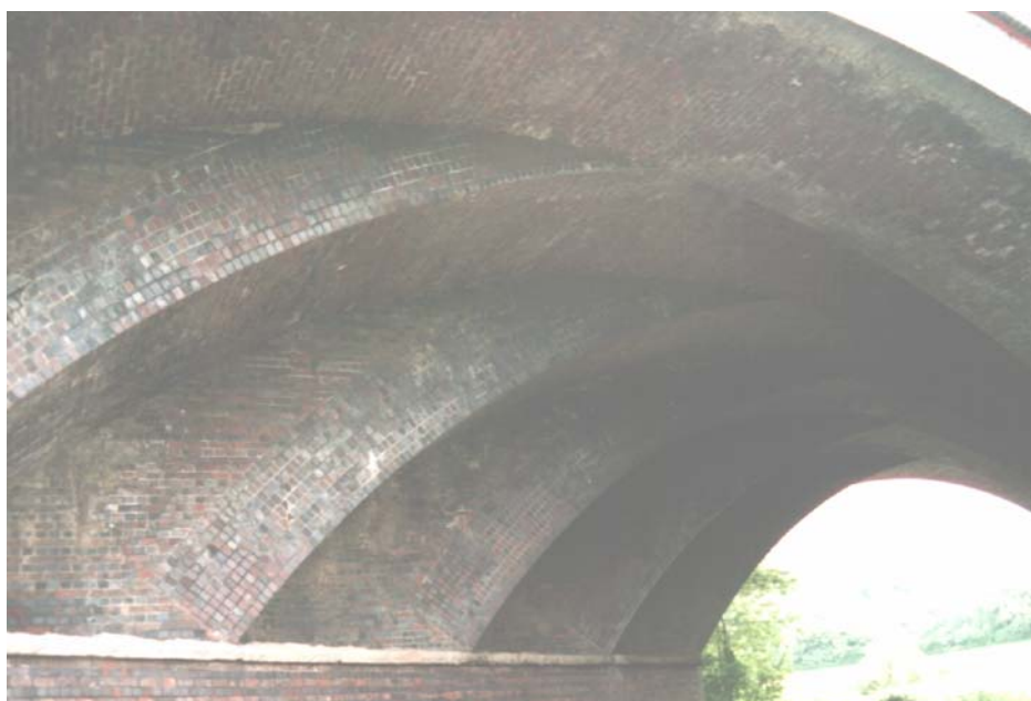
Detail of the bridge near Somerton. A succession of staggered arches – there's modelling challenge!
